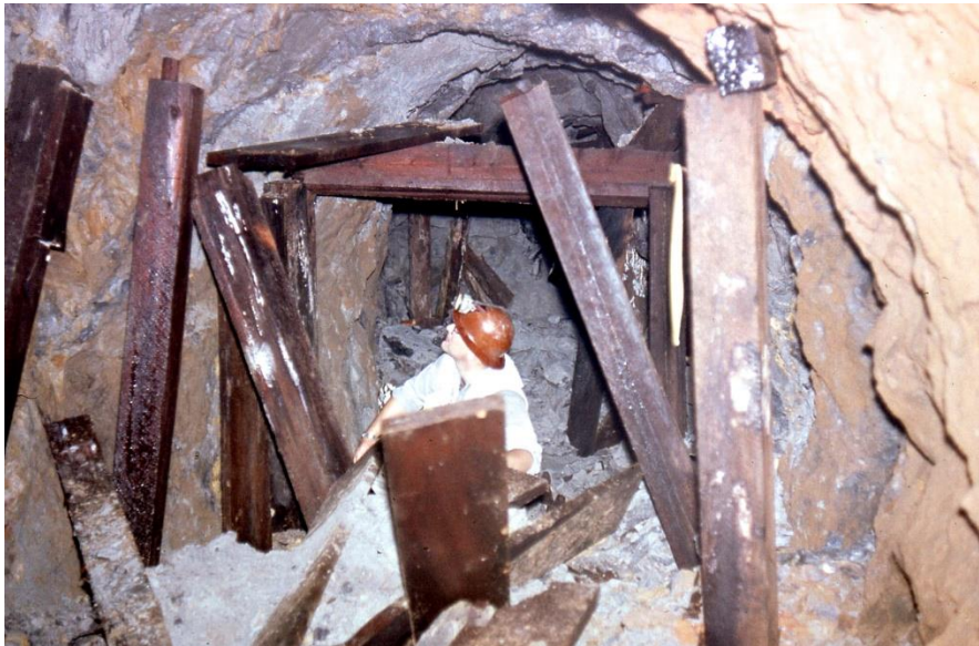
Collapsed support timbers in #3 level
